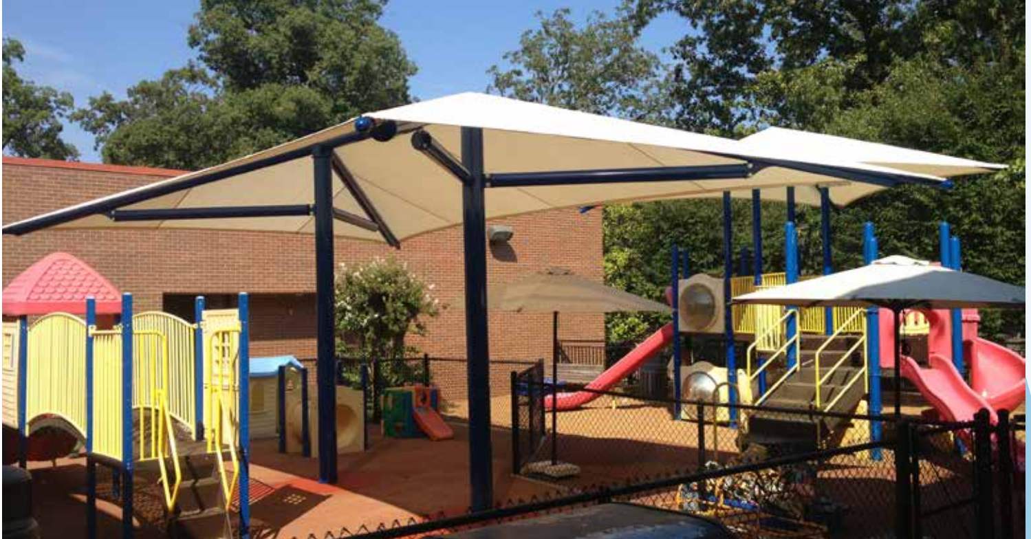
Frame will be made with square or rectangular steel tube.
